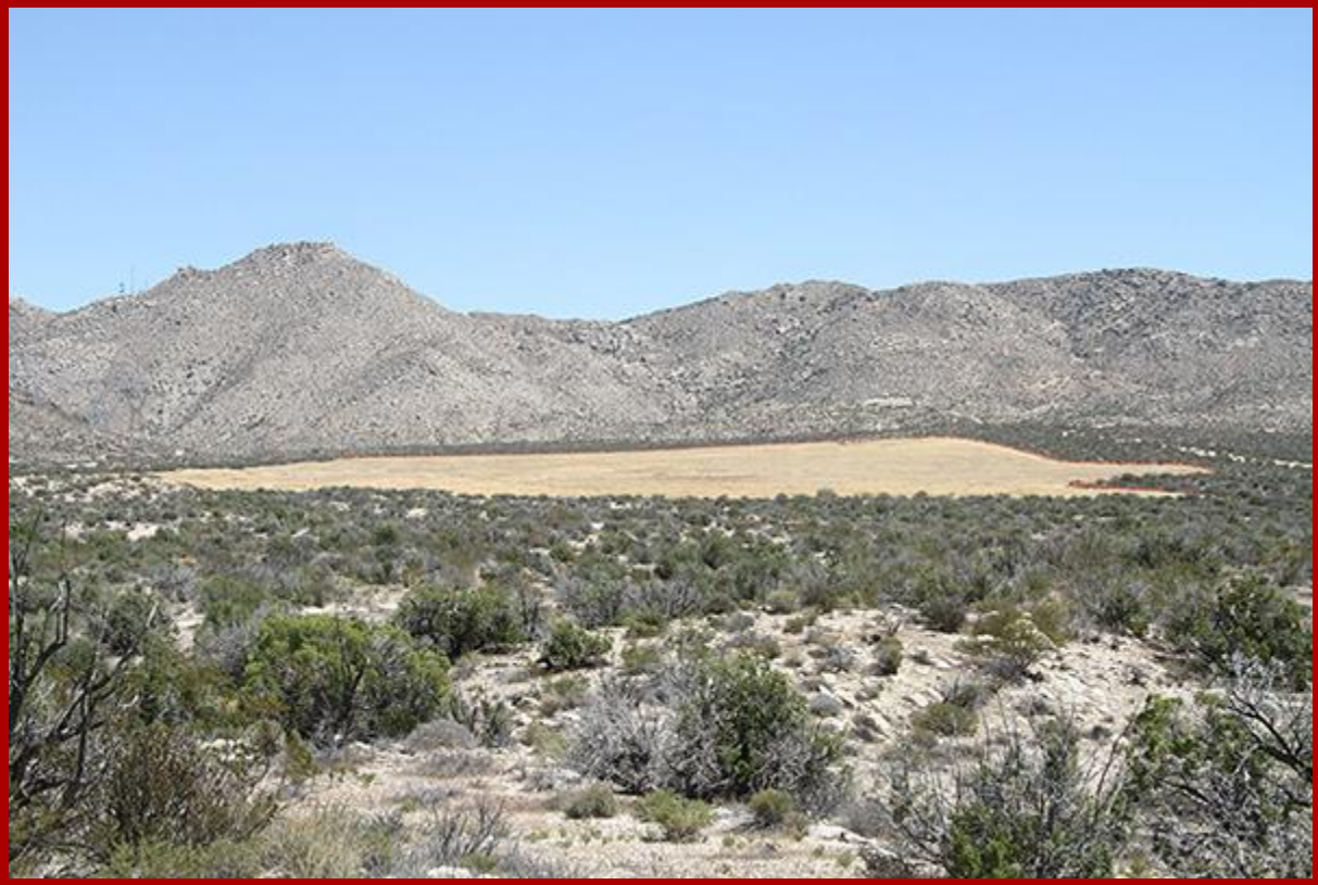
Fig. 20 Site clearance for construction of the Eco Substation.
