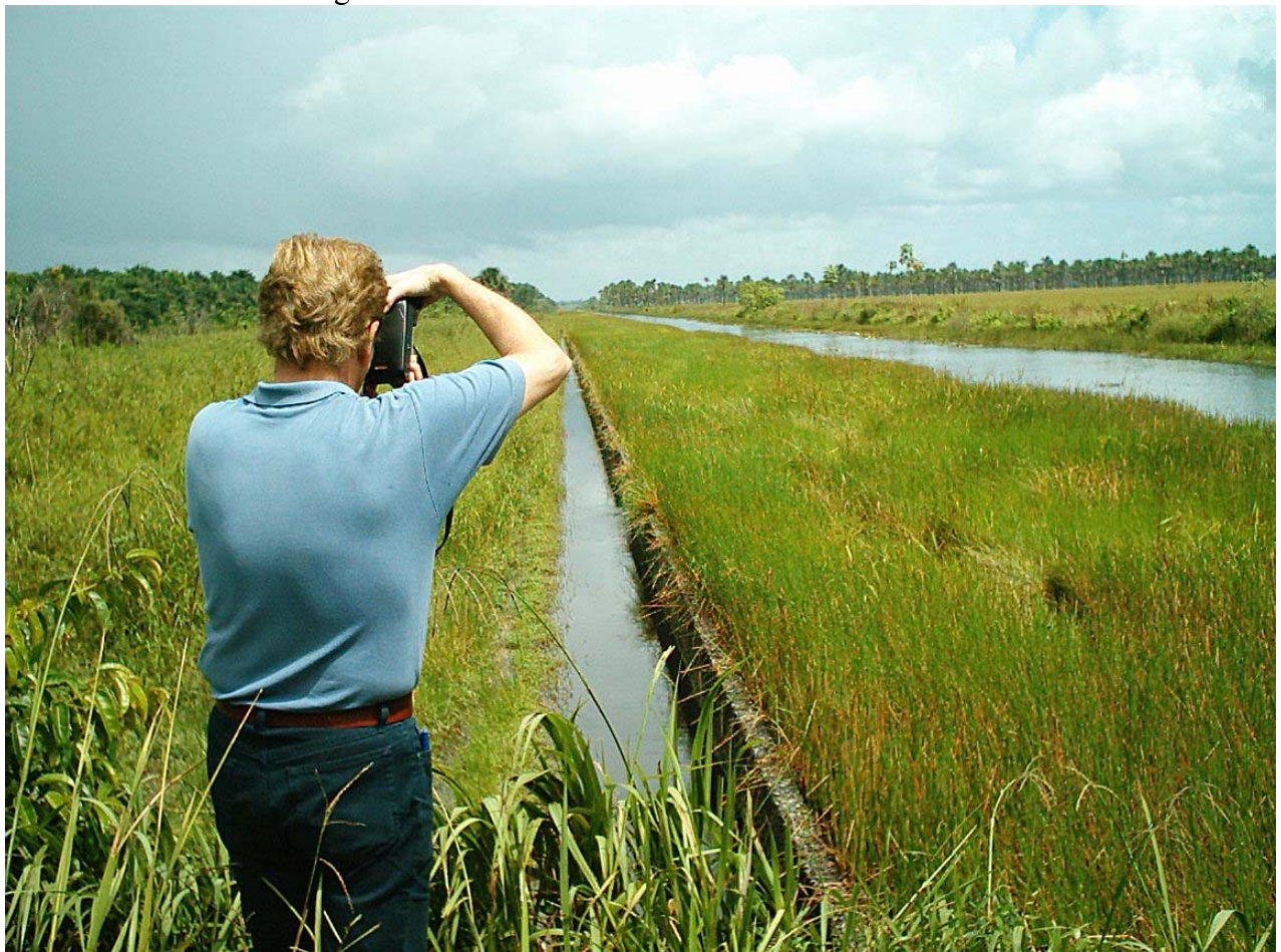
Figure 4.22 The 8000 ft weir
