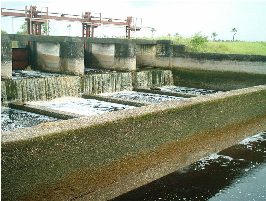
Figure 4.21 Waramia sluice from downstream
