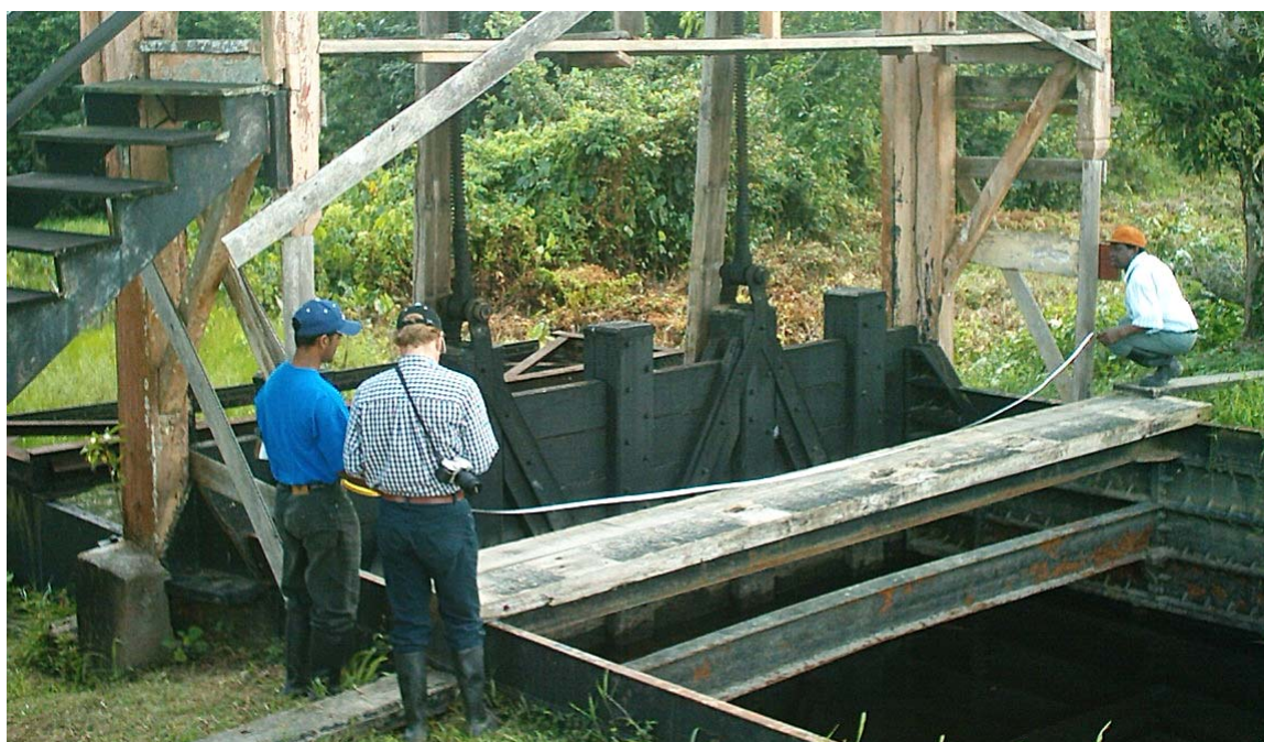
Figure 4.11 Lama Small Sluice
