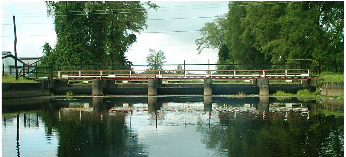
Figure 4.7 Land of Canaan Sluice
