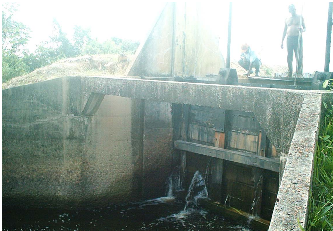
Figure 4.10 Lama Big Sluice
