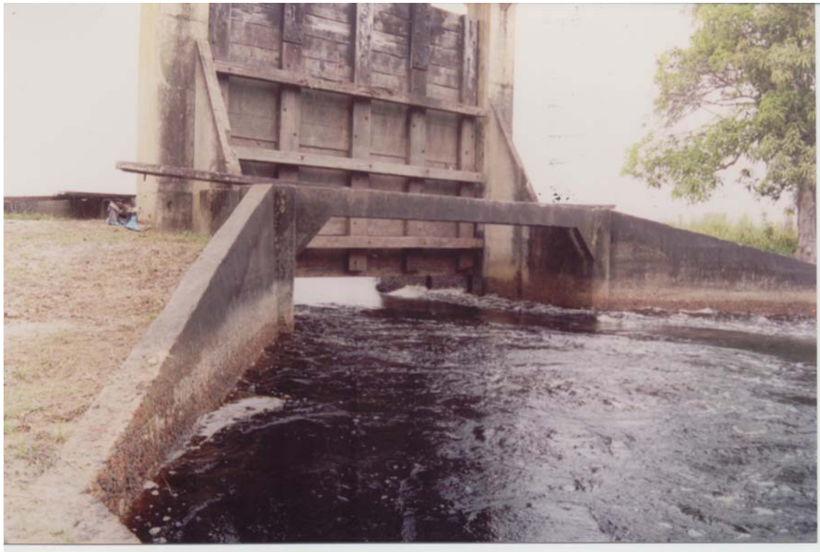
Figure 4.9 Maduni Sluice view from downstream, May 2005
