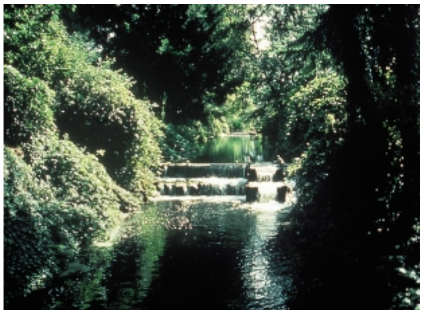
Figure 8.28: Grade control structure. Control measures can double as habitat restoration devices and aesthetic features.
