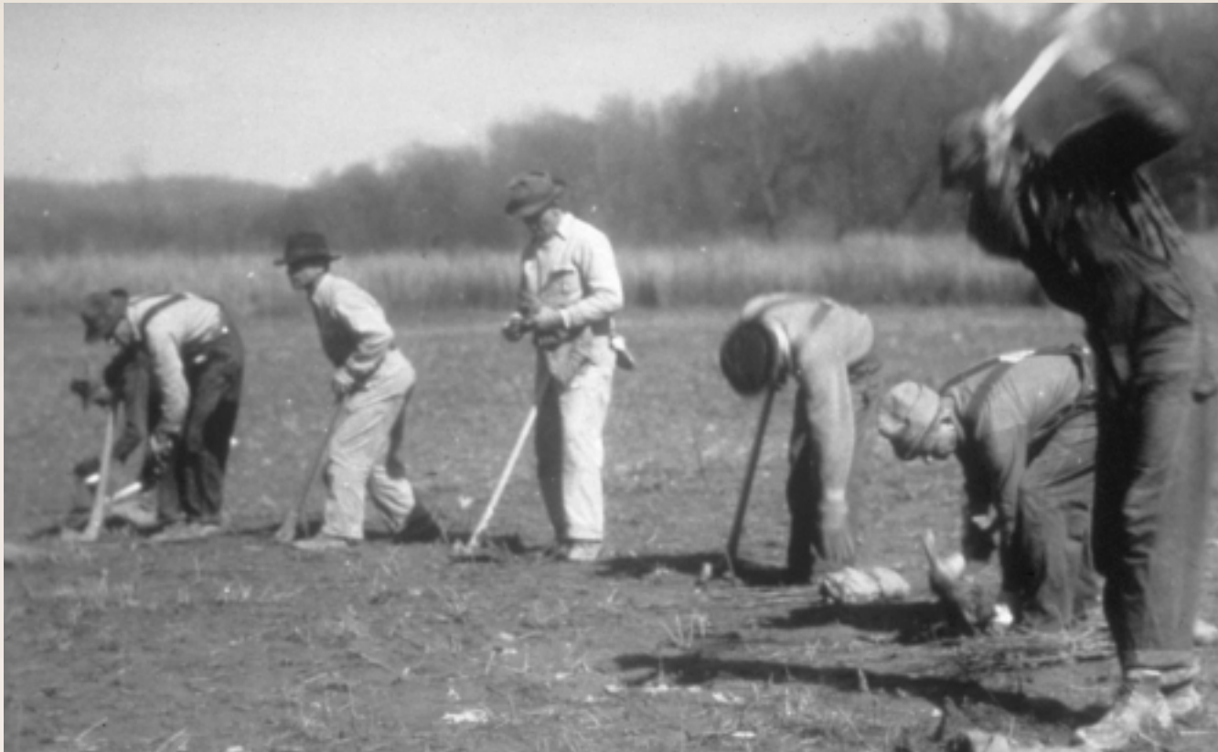
Figure 8.13: Kentucky Reservoir watershed, 1943. Planting abandoned farmland with trees.
